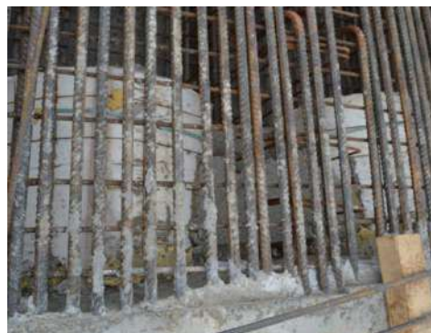
Figure 9. Deck slab reinforcement
