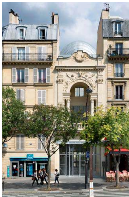
Figure 1. Pathe Foundation, Renzo Piano, Paris, France: Gobelins Theater Façade
