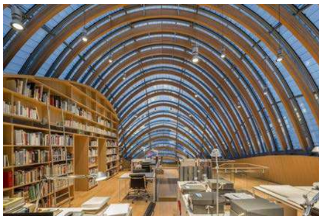
Figure 5. Pathe Foundation, Renzo Piano, Paris, France: Combination of wood and steel in interior (8)
