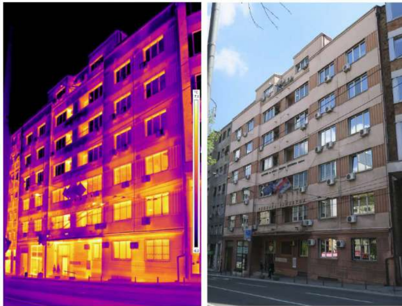
Figure 1. Thermal imaging and photograph of the street facade of the building of the City Municipality of Palilula. The image clearly shows heat losses in horizontal reinforced concrete cerclages as well as beams over windows. No vertical reinforced concrete elements are observed
